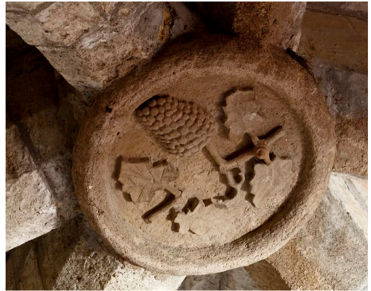
15. Decorated vault keystone in the Tour du Sel
